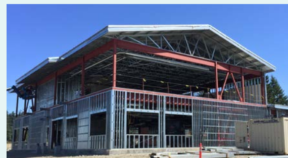
PHOTO: NORTHWEST PARTITIONS, INC
